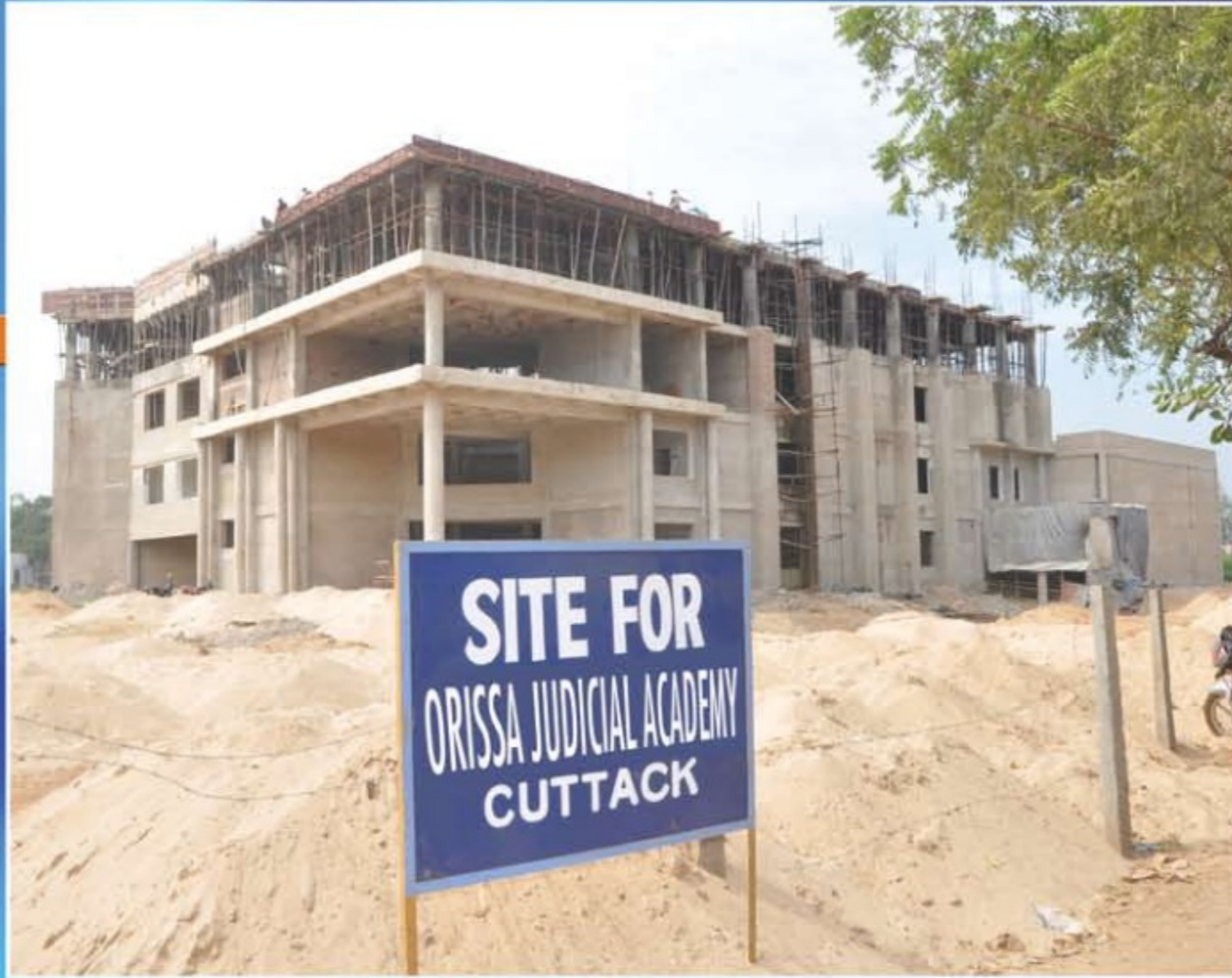
Frontal view of Orissa Judicial Academy under construction
