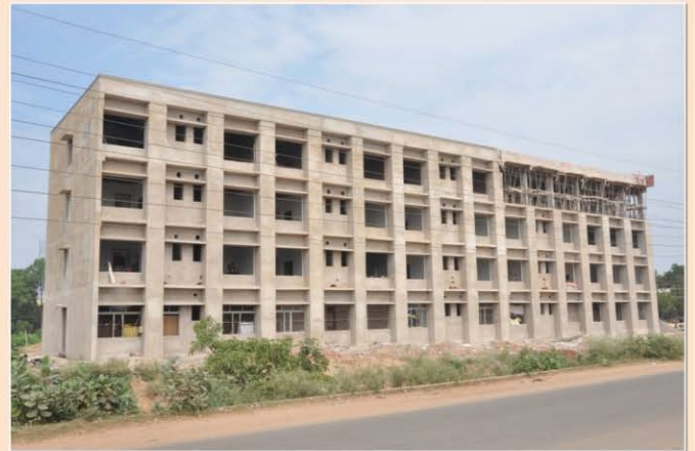
River side view of Orissa Judicial Academy under construction.
